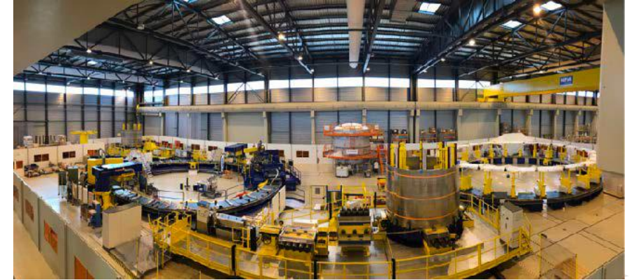
Poloidal Field coils under construction
